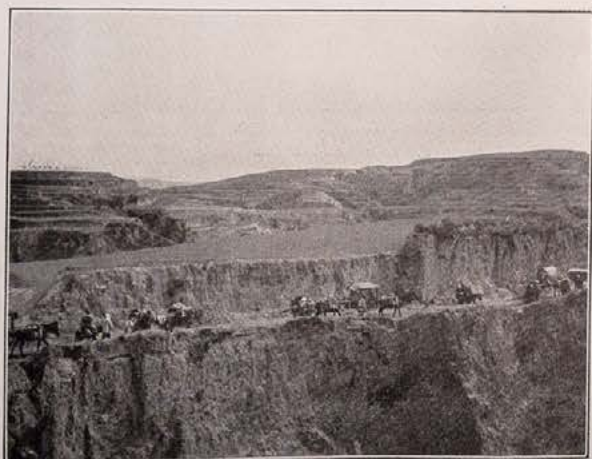
DANGEROUS LÖESS ROADS.
